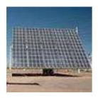
Amonix – has developed **High Concentration Photovoltaic** (**HCPV**) power generation systems for large commercial and utility scale applications offer significant cost savings by using inexpensive flat, plastic Fresnel lenses to concentrate sunlight approximately 500 times. The Amonix high-concentration silicon solar cell holds the world record for the performance of a cell manufactured in a commercial environment. (26.5%
