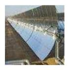
**Flagsol** has their New Solar Collector which are a new line of parabolic trough collectors that will reduce costs by 15%-20%. Flagsol is showing that solar thermal energy costs-per-Kw can match or beat cost-per-Kw for coal or fossil fuels. **http://www.flagsol.com**
